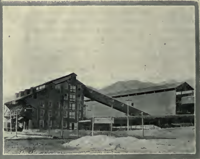
SINTER MACHINE BUILDING, LOOKING NORTHWEST.
